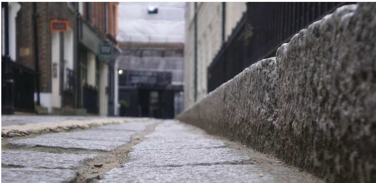
Took's Court, kerb detail
